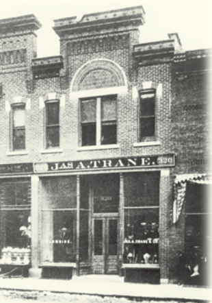
Trane Storefront La Crosse, Wisconsin 1891
