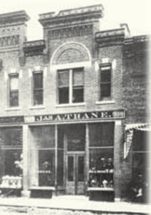
Trane Storefront La Crosse, Wisconsin 1891
